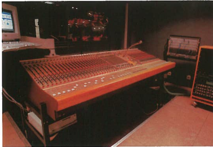
The 48-input Cadac J-Type console, fitted with motorised faders and comprehensive automation facilities.
